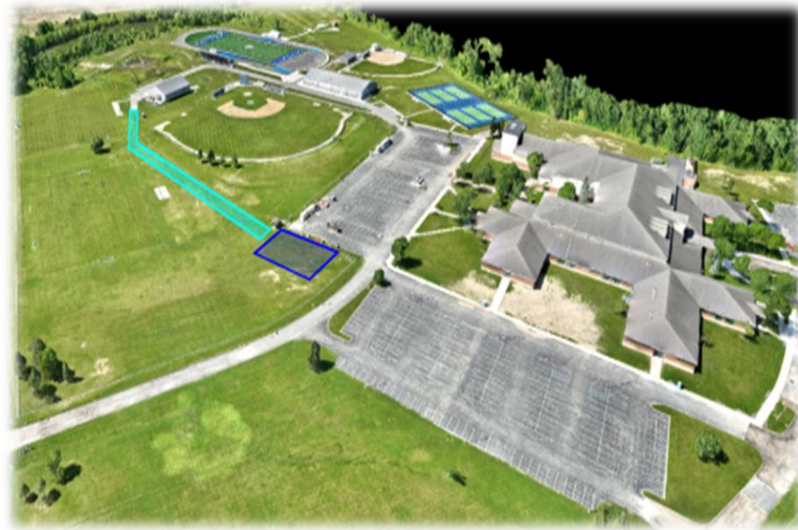
Location of New Administration Building and Road to the Water Treatment Area
