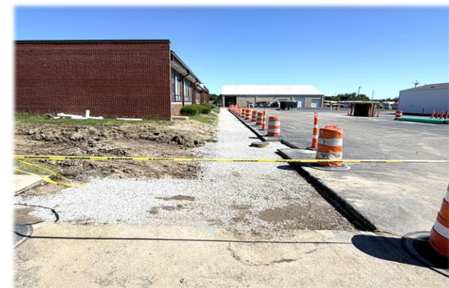
Prep for Concrete Sidewalk
