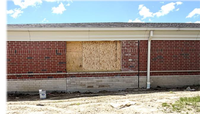
Masonry Repair on Classroom Exterior
