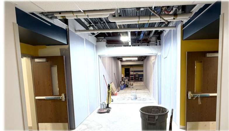
Corridor Connecting Existing Building
