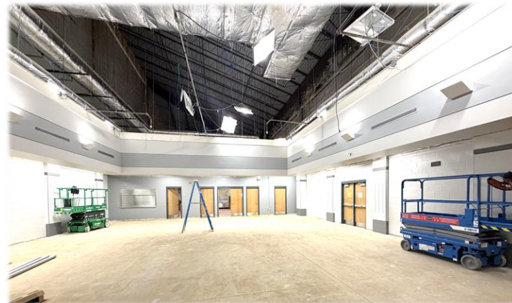
Painting and Ceiling Replacement
