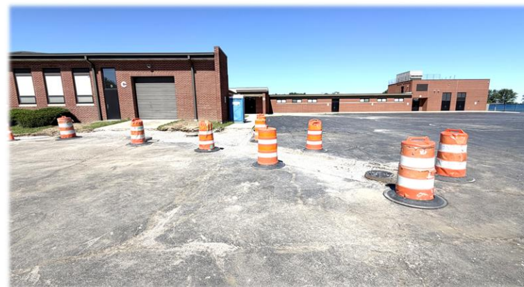
Masonry Repair - Classroom Window
