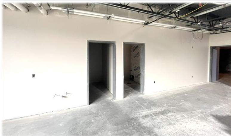
Classroom Restrooms and Storage Room
