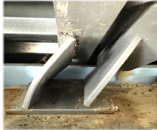
Existing Steel Roof Joist Condition
