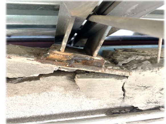
Existing Steel Roof Joist Condition
