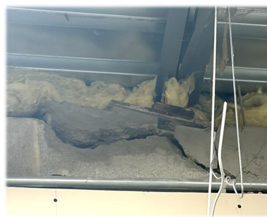
Existing Stele Roof Joist Condition
