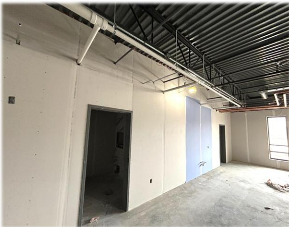
Classroom Restrooms and Storage Room
