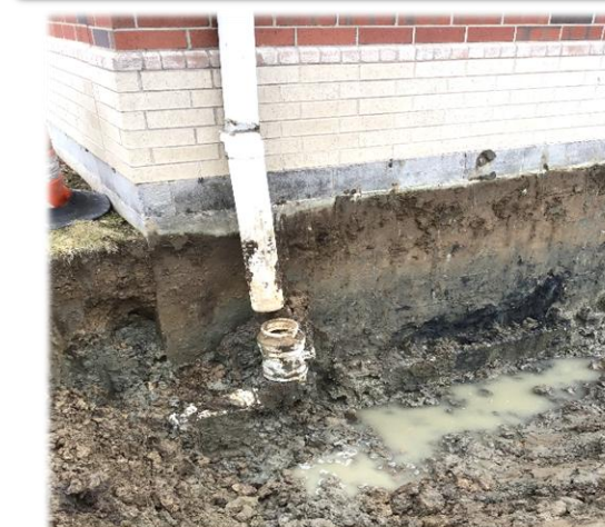
Excavation for Helical Piers
