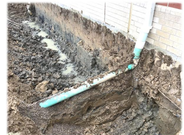
Excavation for Helical Piers
