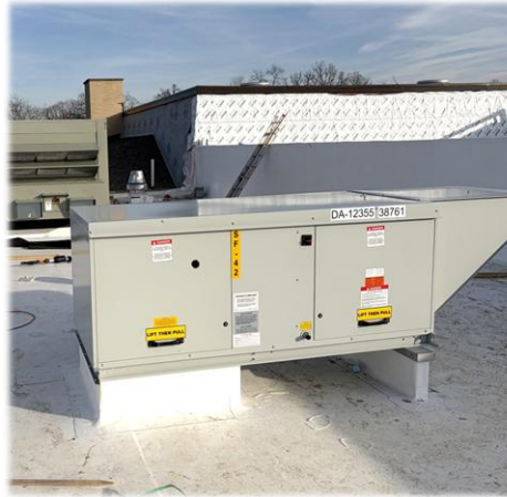
Roof Top HVAC Units Set on the Roof
