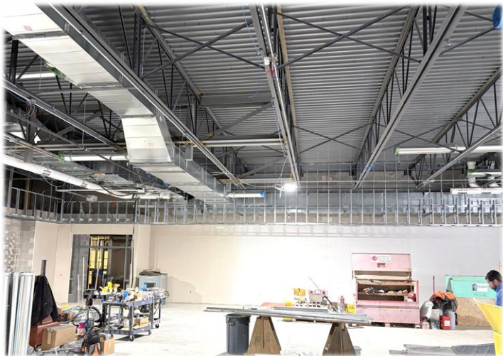
Cafeteria Painting and Ductwork Installation
