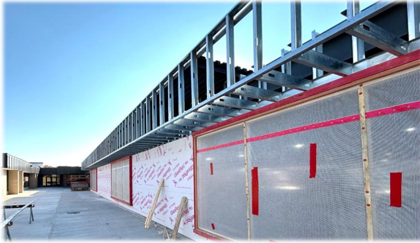
Soffit Framing on the Courtyard Side
