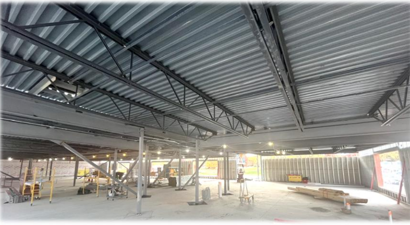
Structural Steel Joists and Metal Decking
