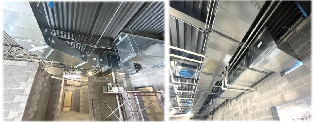
Ductwork Installation
