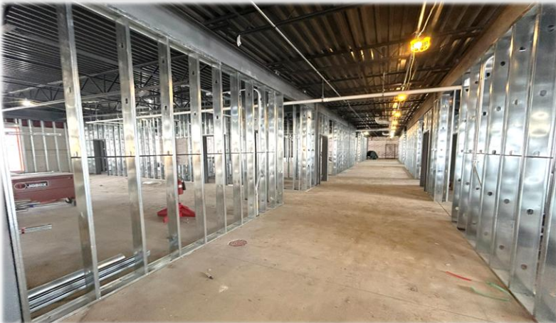
Framing Metal Stud Walls in the Corridor
