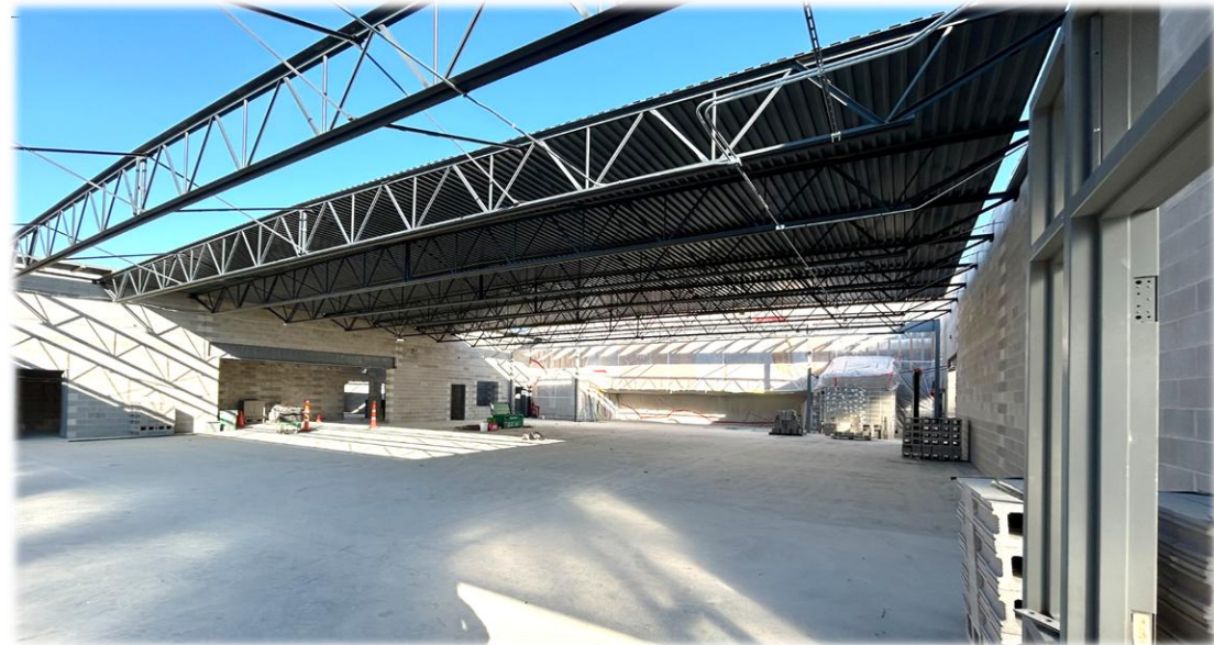
Kitchen Structural Steel and Roof Decking
