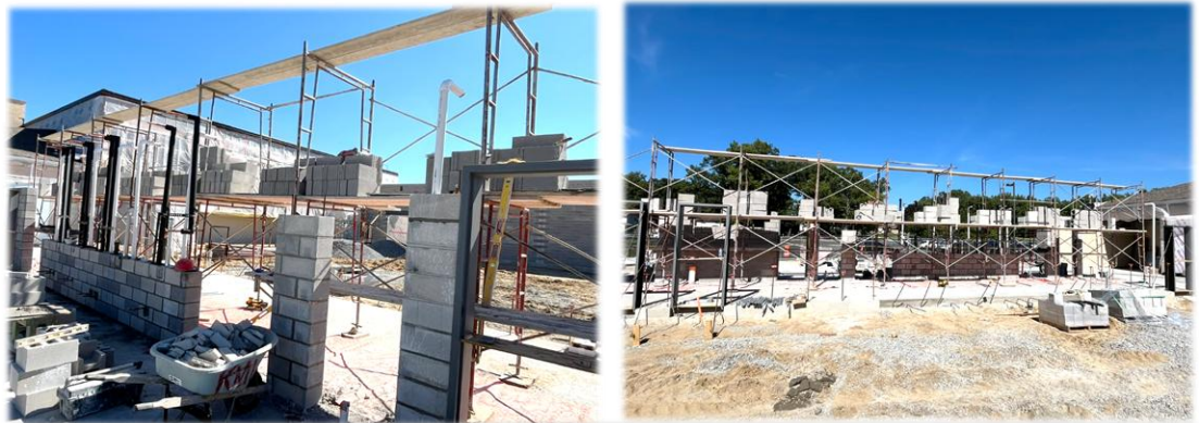
Exterior CMU Walls and In-Wall Plumbing/Electrical Rough-Ins
