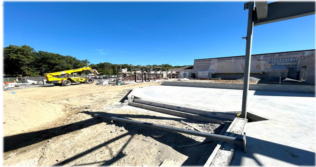
Northwest Entrance/Exterior CMU Walls
