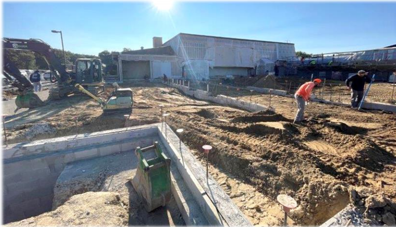
Backfilling the Footings & Foundations for the Kitchen/Café Addition
