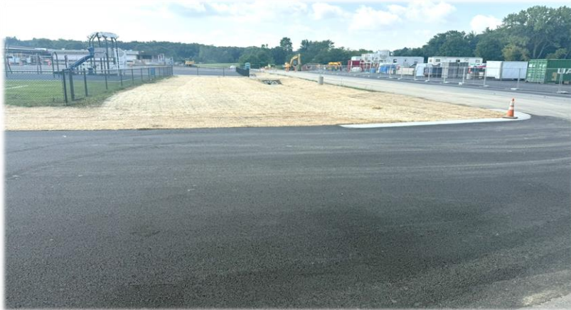
Grass Seeding and Asphalt Paving
