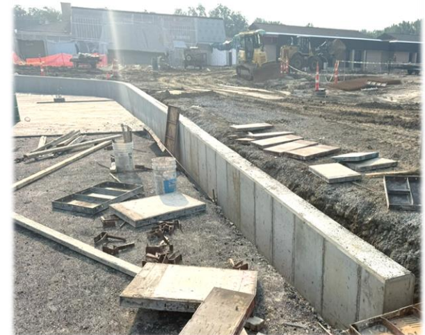
Concrete Retaining Wall along Hard Play Area & Sidewalk
